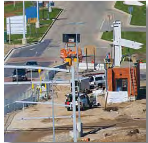
Work continues on the gateway entrance plaza along Oostema Blvd.
